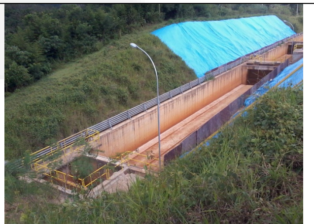
F6 - talude a recompor
